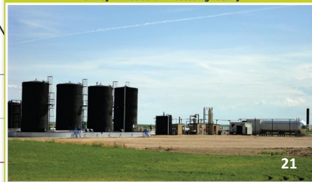
Smiley Whiteside Oil Processing Facility
